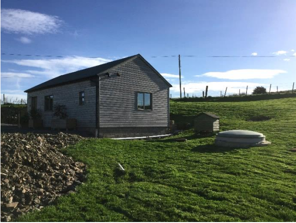
Side of wooden insulated building, temporary meter box and sewage treatment plant
